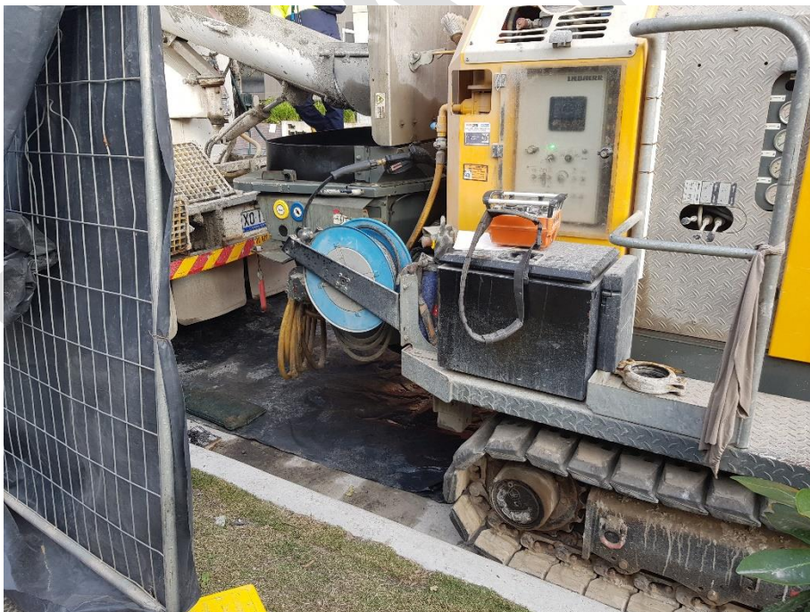
Photo 12: Sediment controls in place under the concrete truck.
