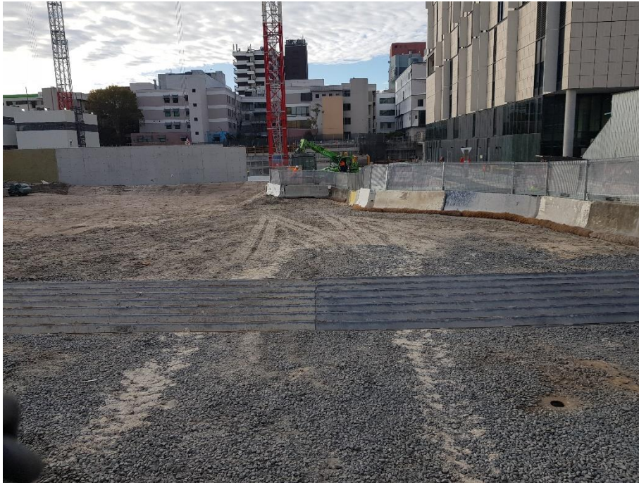
Photo 15: Rumble grid at the gate entrance to the southern end of the property that was still under the control of John Holland Group on Botany Street, looking towards the east.
