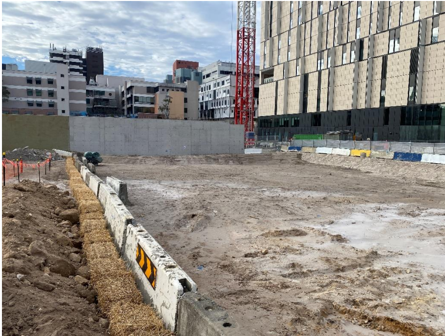
Photo 9: View to the east across the southern portion of the property that remained under the control of John Holland Group prior to its handover. Flood mitigation measures at the southern end and sediment controls along the boundary.
