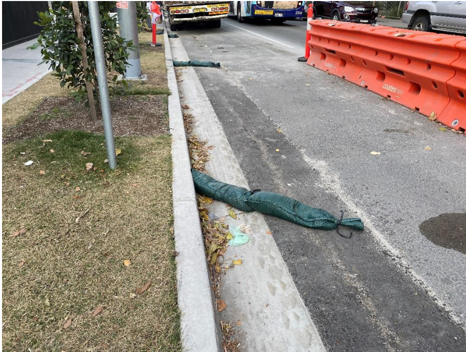
Photo 13: Sediment controls in place along Botany Street, looking towards the south.
